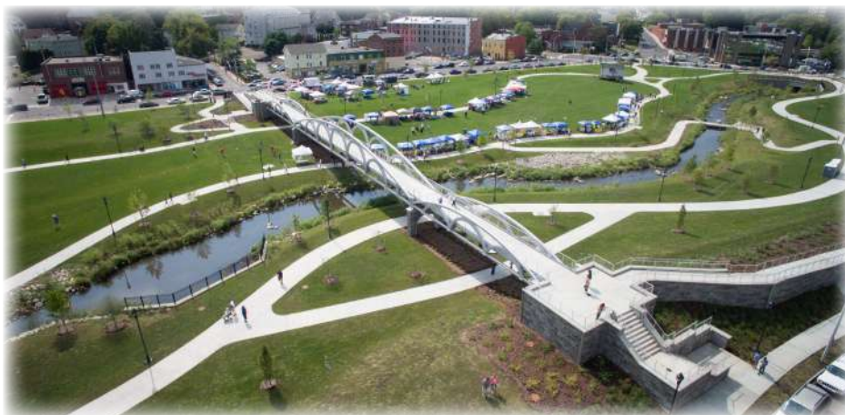
Above is an aerial view of Meriden Green & Silver City Bridge
